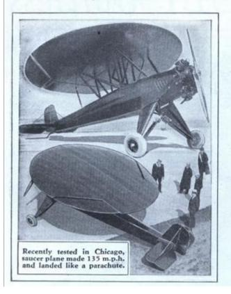
FIRST cousin to the autogiro, a new circular-wing airplane recently tested in Chicago is so simple in operation that one who has never been off the ground can learn to fly it in thirty minutes, according to the inventor.
