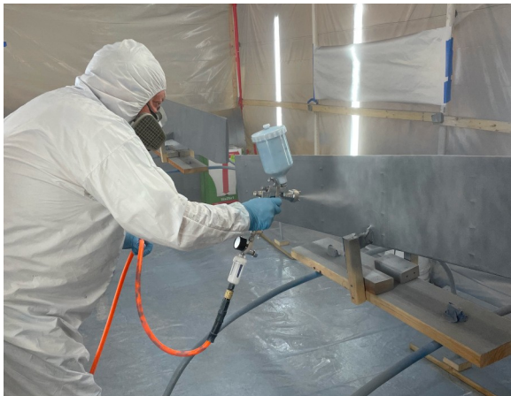
Kim Johnson applying primer.
