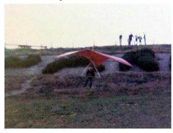
I also built and flew a bamboo hang glider called a Batso that we first saw in Popular Mechanics. We used to jump off "Mount Centennial" which was really the garbage hill in Etobicoke. We also used to tow it behind a mini bike! When we crashed it my Dad would sleeve it back together with aircraft aluminium.
