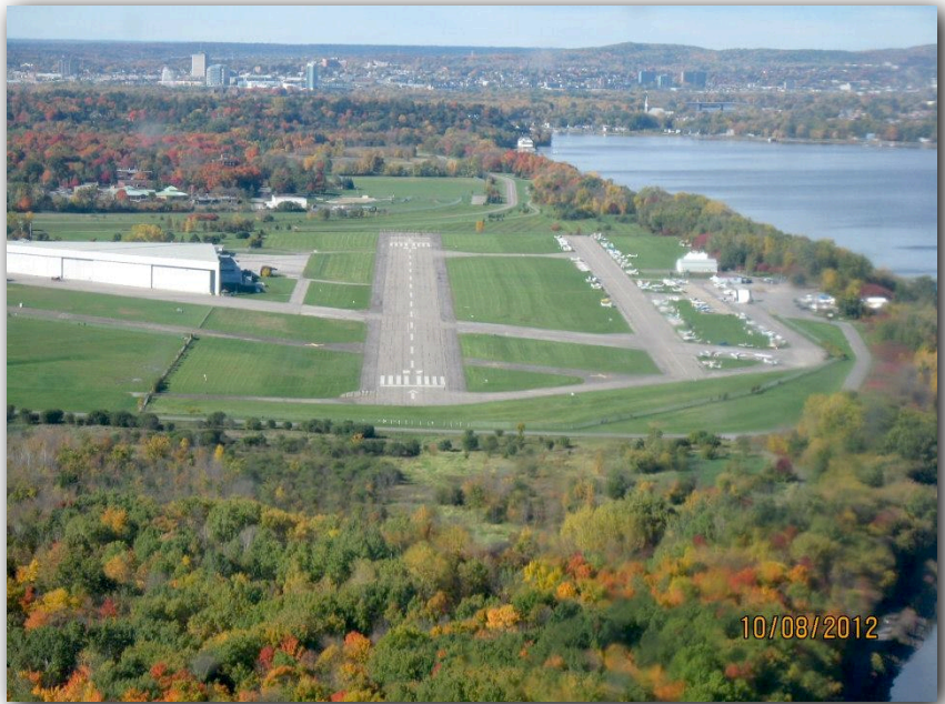
DPZ on Approach to Runway 27 in Rockcliffe
