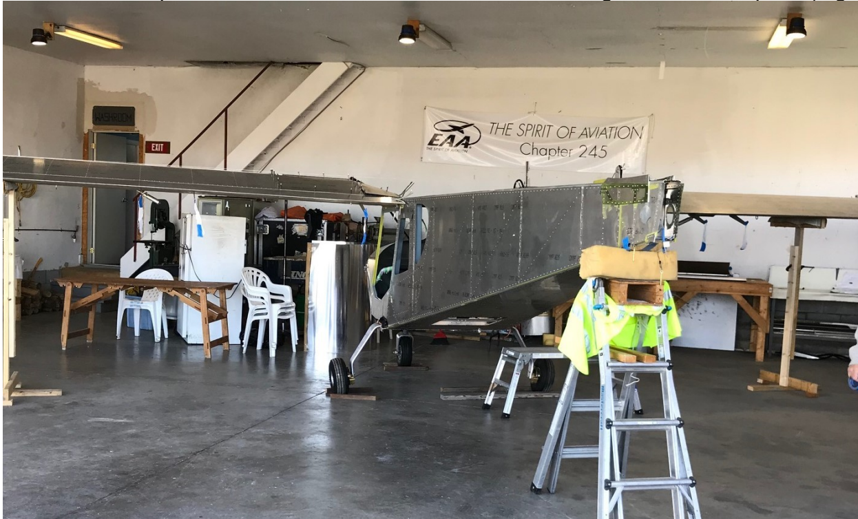
Figure 2. The wings are installed, perpendicular to the fuselage centre and with dihedral set. The wing stands were left in place and their respective heights were clamped and screwed to hold them secure.
