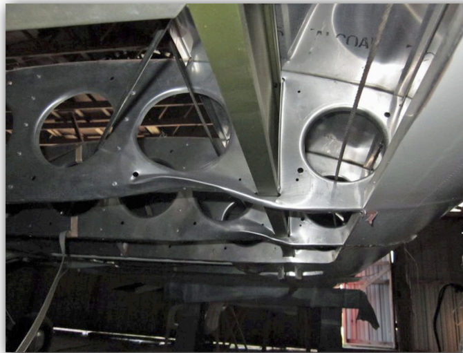
Photo 2: Interior Rib Damage
