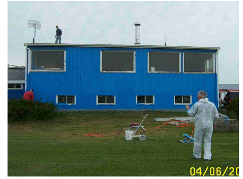
Cary on the roof replacing shingles
