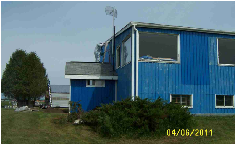
The painting continues and the septic crew makes progress
