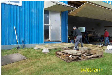
Russ Robinson, Grantley Este and Steve worked on the front steps
