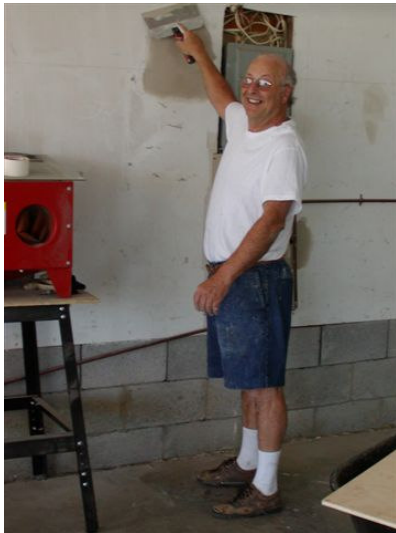
Photo 1 Dick repairing the hangar wall
