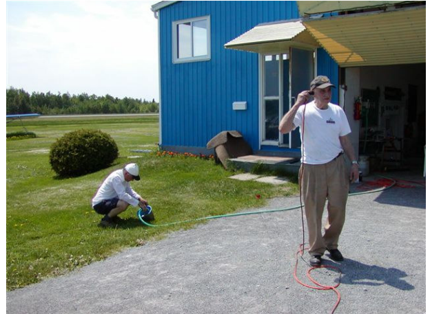
Photo 4 cleaning up after painting
