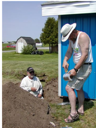
Photo 2 Grant, Martin and Cutis insulating the drain from the recent addition
