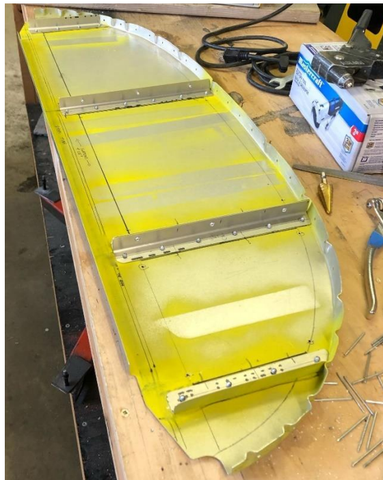
Figure 2. Three subpanel bays are separated by L-angle stiffeners prior to cutting out the openings.
