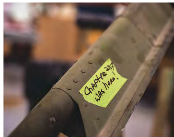
No detail is too small—or too inaccessible—when it comes to a restoration like this one.
