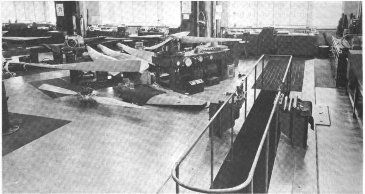
Figure 13.10.—Propeller shop balance pit.
