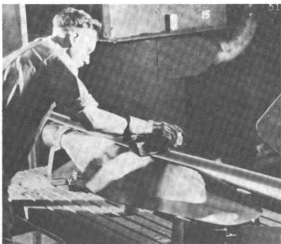
Figure 4.19.—Belt grinding hollow blades.
