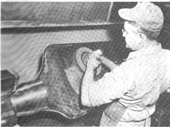
Figure 4.12.—Propeller blade finish grinding
