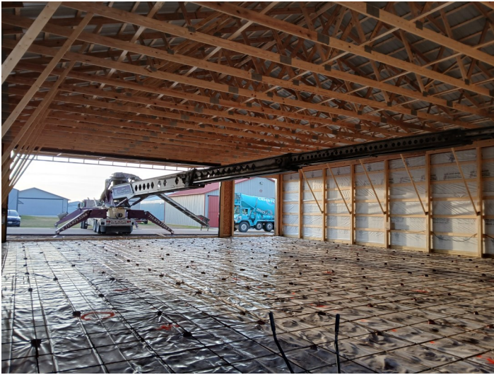
Inside Scott's new hanger and pouring cement for the floor.
