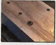
4. You aren't trying to drill all the way through the rivet shank—just deep enough to separate the head from the shank. If you feel that you are drilling into the surrounding material, stop!
