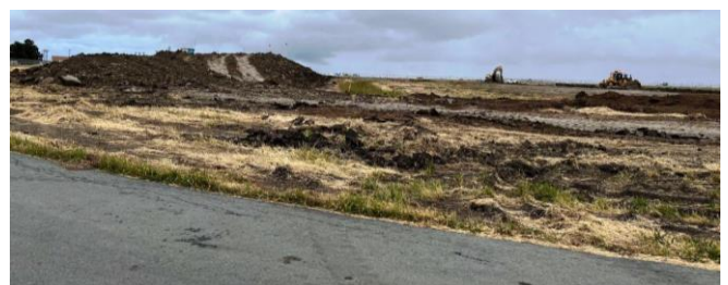
Grading underway for San Diego MetroPark near Old Charlie. 4/23
