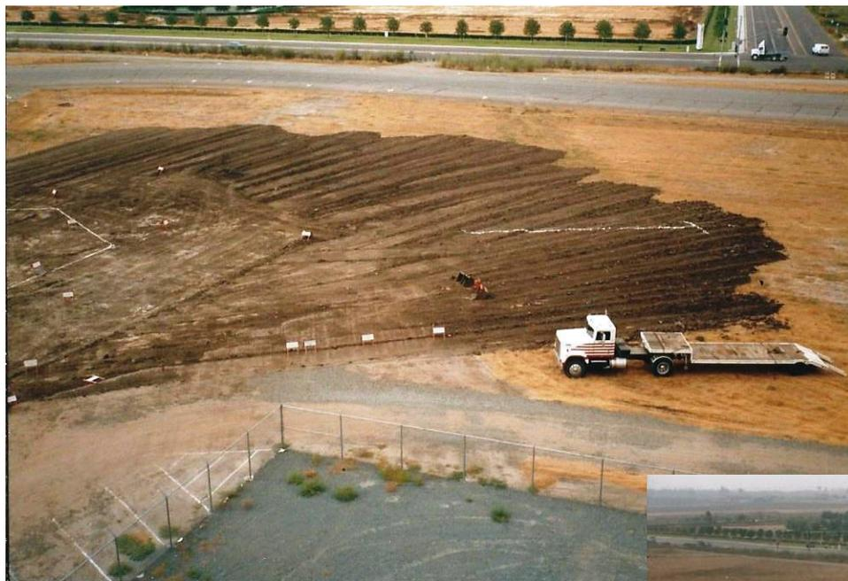
Backhoe trenches for utility and drainage in preparation for building Hangar 3
