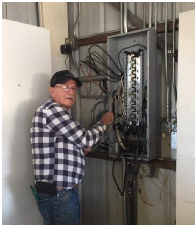
Ron Shipley looks up from replacing the Main Electrical Panel in Hangar 1.
