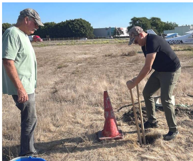
Gary List and Rich Allison install a new tiedown pier on the flight line to secure Rich's Skyhawk.
