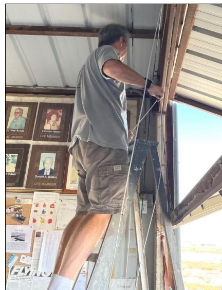
Nigel Worrel installs our new electric winch on the Hangar 1 Door.
