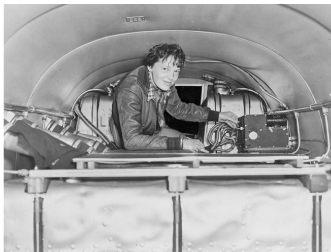
Amelia Earhart leans over the additional fuel tanks installed in the aft cabin of her Model 10E Special. The fuselage tanks, totaling over 750 gallons, took up all the space between the cabin door and the cockpit, requiring the crew to crawl over them to enter the cockpit.
