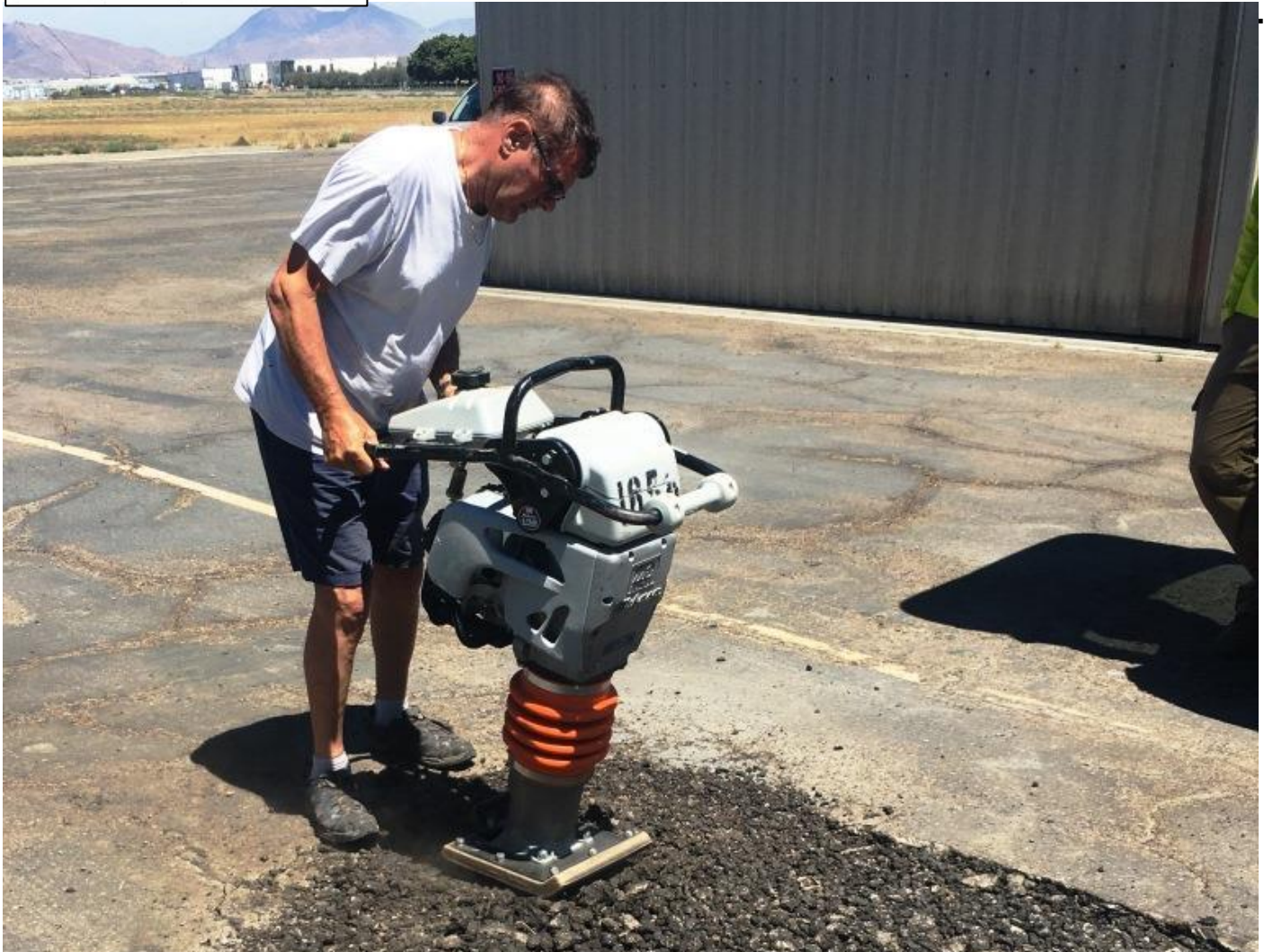
Trevor Pearson tamps down asphalt to repair damage to the EAA-14 ramp from a heavy vehicle.
