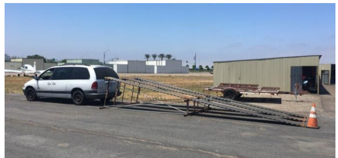
Loading ramp for the Katana. Ryan constructed this ramp from scaffolding and landing mats donated by the Border Patrol. We always knew that they would come in handy.
