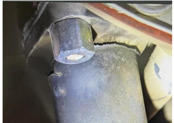
Exhaust pipe crack, identified through anomalies in CHT data.
