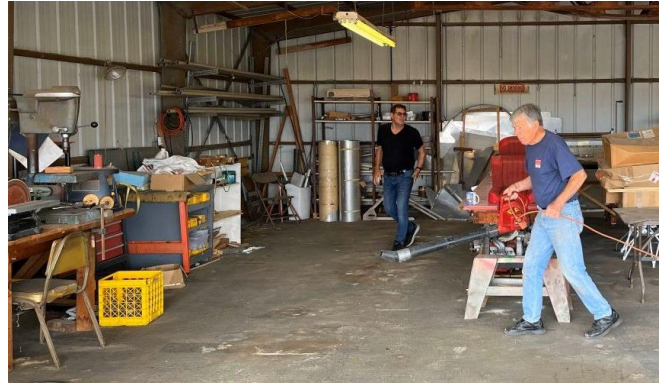
Starting a week ahead of time, volunteers cleaned up Hangar 2 in preparation for the Build-a-Box workshop. 6/1
