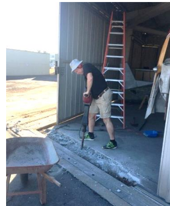
Chapter President Gene Hubbard uses the Chapter jackhammer to remove damaged Hangar 3 door tracks. You didn't know that we had one, did you? 12/4
