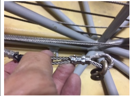
Adjustment of cable length
