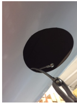
It will fit here in this inspection hole
