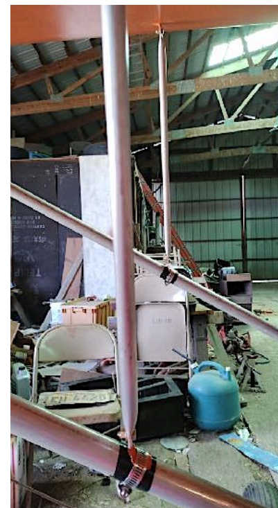
Installed jury struts
