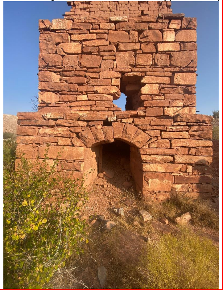
Old smelting furnace at Grand Gulch copper mine.
