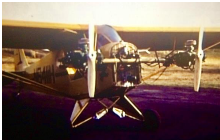
Modified Piper J-3 Cub with 2, 40 horse power two cycle air cooled engines, fabricated by Don Sullivan, mid 1960s
