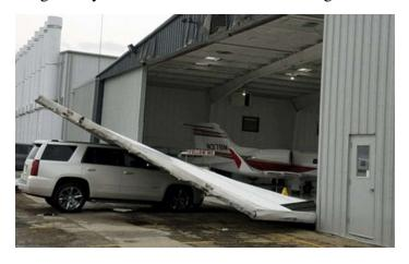
This rolling door section dropped off the track. Severe storms can cause even heavy doors to lift off the track and fall onto your aircraft. In your storm prep, a couple of chains at the top can save you from real heartbreak if the storm should derail your door. Notice the compression of this car's suspension; imagine getting caught under the falling door.
