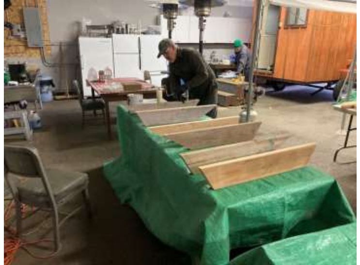
Rod Case applies primer to boards pre-cut by Jim which will be assembled into replacements for the deteriorated sections of the segmented circle.
