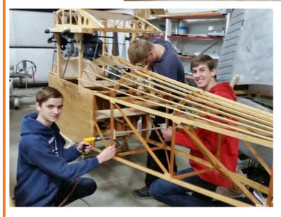
Starting to install the control mechanics.
