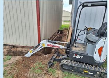
are squeezed with tremendous pressure during the winter. To fix this, I've excavated below the frost depth (~52") around the perimeter and added an insulative frost barrier that will keep the clay below the building from freezing. I'll also finish insulating the building interior and ceiling and
