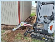
are squeezed with tremendous pressure during the winter. To fix this, I've excavated below the frost depth (~52") around the perimeter and added an insulative frost barrier that will keep the clay below the building from freezing. I'll also finish insulating the building interior and ceiling and
