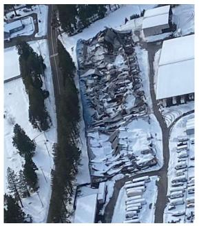
You might wonder, "Can a snow load damage a hangar at Placerville?" The answer is yes, depending on the amount of snow and whether one attempts to open the hangar door. One tenant noted the roof truss depressed when the folding door was opened and could not be closed again. I was not allowed out of the vehicle, so I stood on the running board and shot the picture below.
