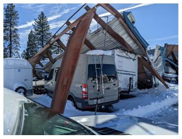
The picture below shows the windshield of a large class A motor home demolished by the twisted steel beams and snow laden roof.
