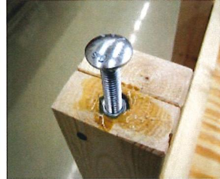
Here we just drilled the hole for the shank of our 1/2-inch carriage bolt. Then drilled a shoulder for the nut. You'll need to use a chisel to conform the hole to the nut and press fit it in. We added a little 5-minute epoxy to keep the nut in place.
