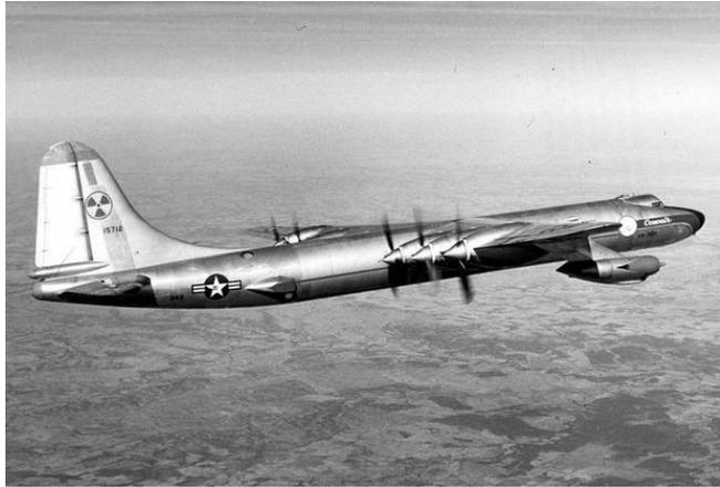
A modified B-36 Bomber became the nation's only flying nuclear reactor in 1955. The plane, which became as the Nuclear Test Aircraft, help explore nuclear-powered propulsion and the effects of radiation on airframes. (U.S. Air Force photo)
