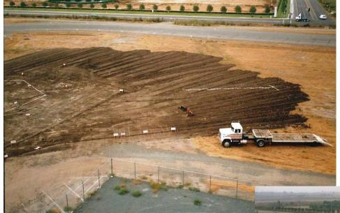
Backhoe trenches for utility and drainage in preparation for building Hangar 3
