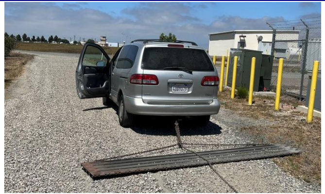
Resurfacing the driveway with gravel donated by F. J. Willert Contracting Company in Chula Vista. Thanks to Gary List for obtaining the donation and to Ryan for constructing the drag and levelling it out.
