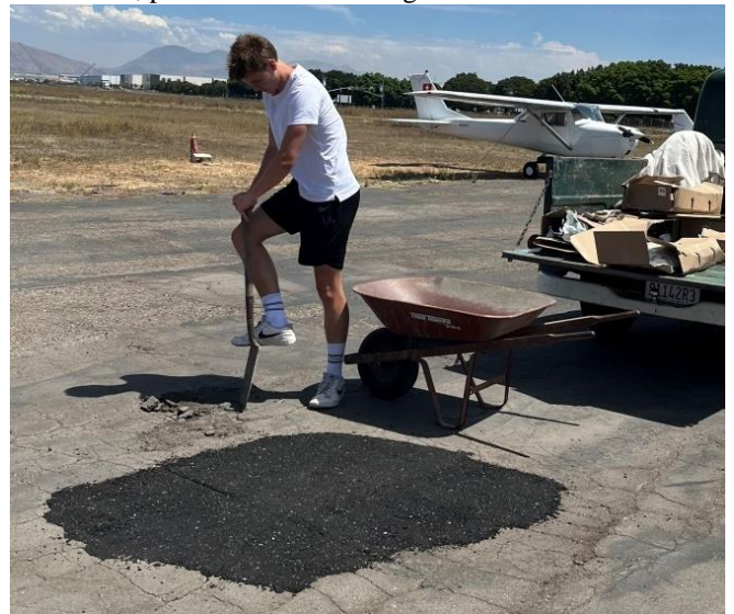
Patching the ramp. A volunteer helps dig out bad sections after getting a flight with Ryan.
