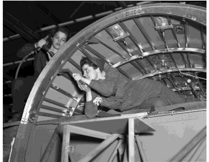
Two women install rivets on the center wing section of a B-24E at the Willow Run Bomber Plant sometime between July 1942 and February 1943.
