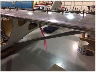
Work progresses! We just finished fitting and mounting the wing struts. In order to do the work, we had to rent a special jig from GlasAir in Arlington, Washington.
