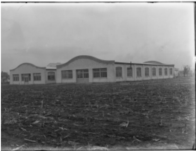
Historical image of the Wright Company factory buildings circa 1911, from Library of Congress.
