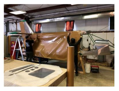
the glue and seal it to the surface while taking time to push it down around every rivet.
